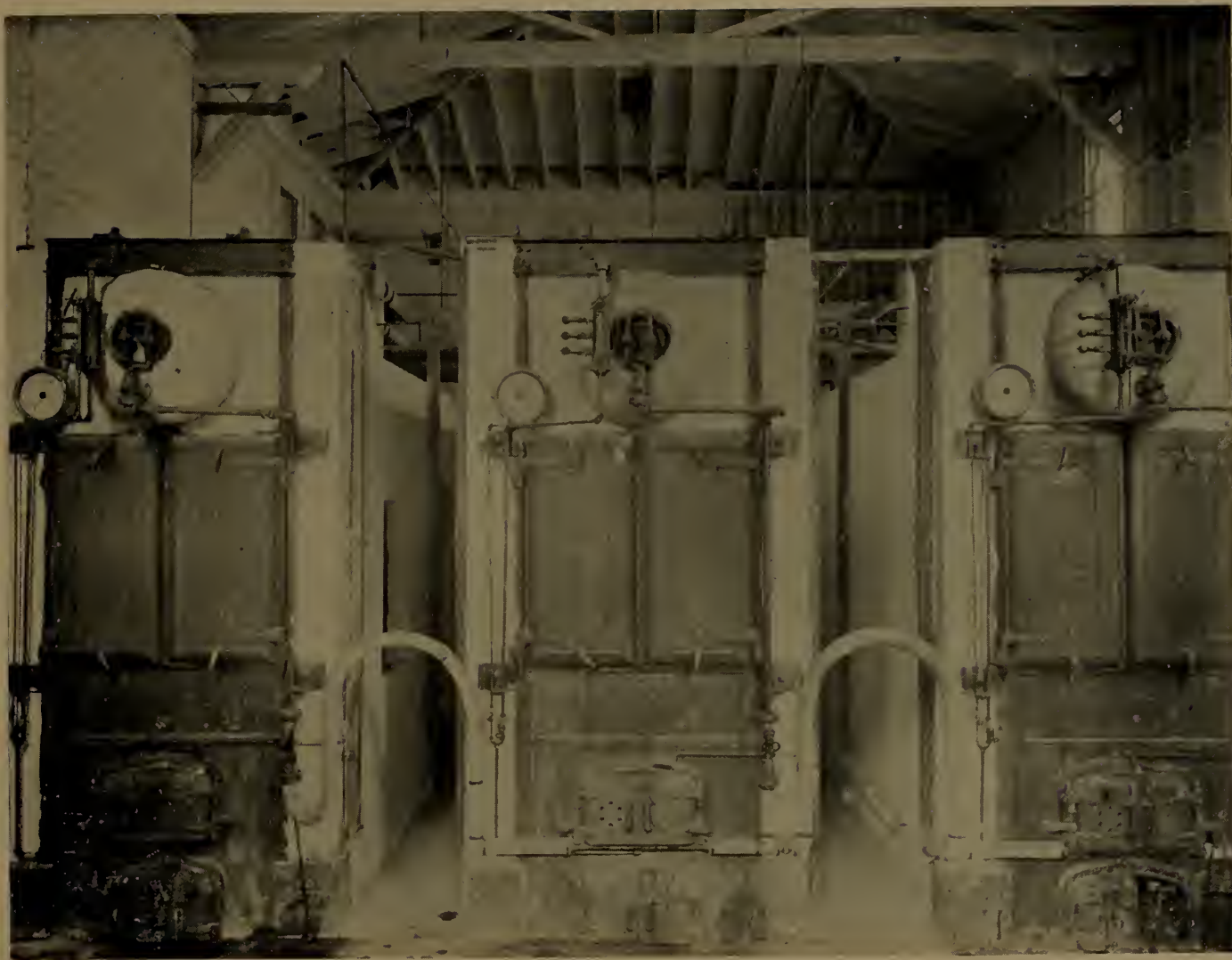
Boiler Room, Sutro Baths and R. R.
