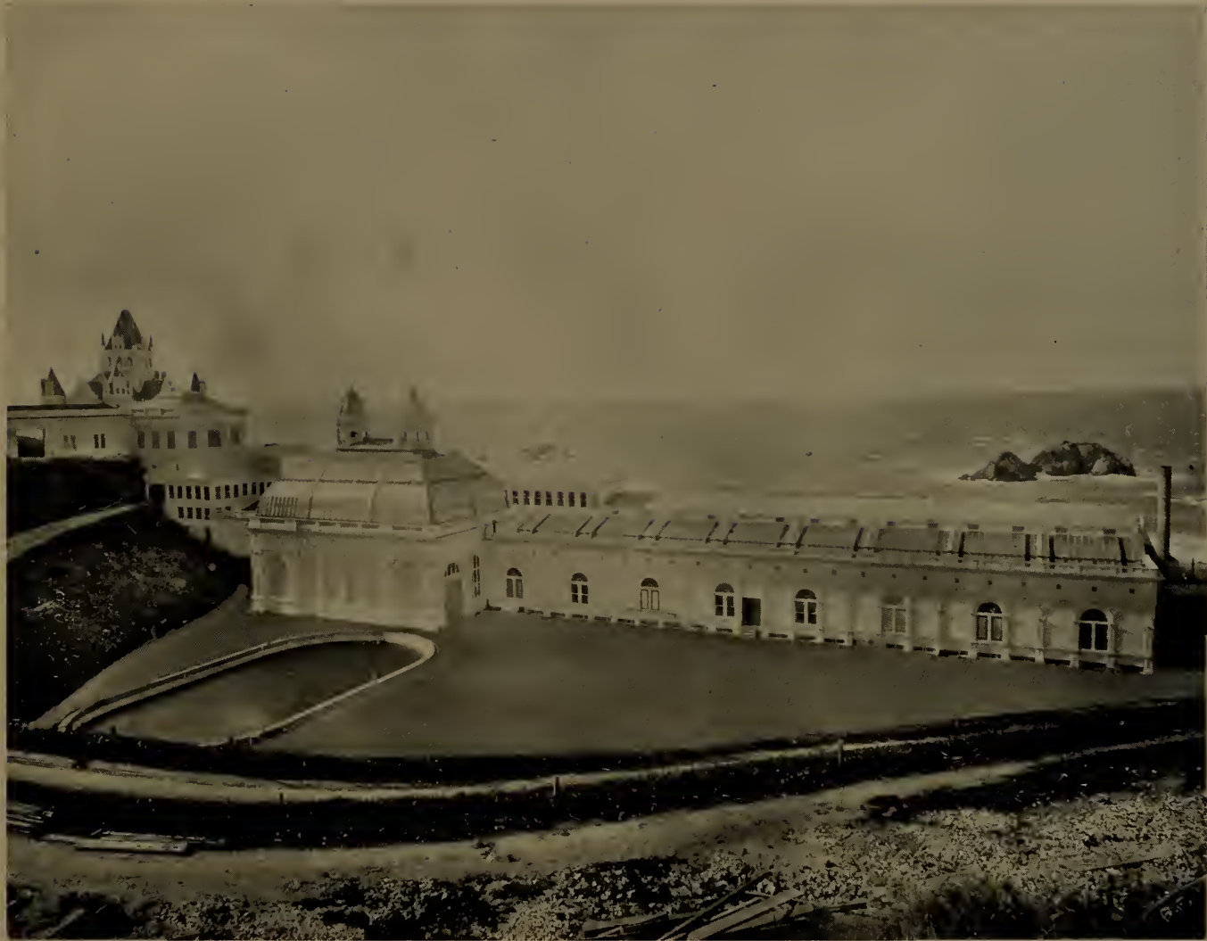
General View Sutro Baths, looking West,
