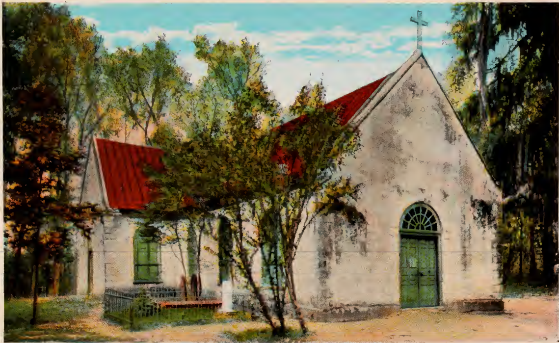
ST. ANDREWS PARISH, BUILT 1706, CHARLESTON, S. C.
